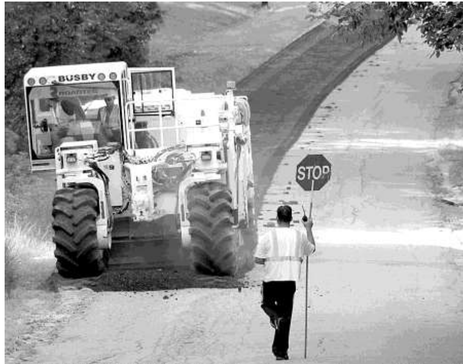
ROAD GRINDING - FR Carroll of Limerick ground sections of Mill Hill Road Aug. 20 in preparation for paving from Hawk Mountain to Passaconaway. The grinder was also used on the Baker Hill section of Mill Hill.
