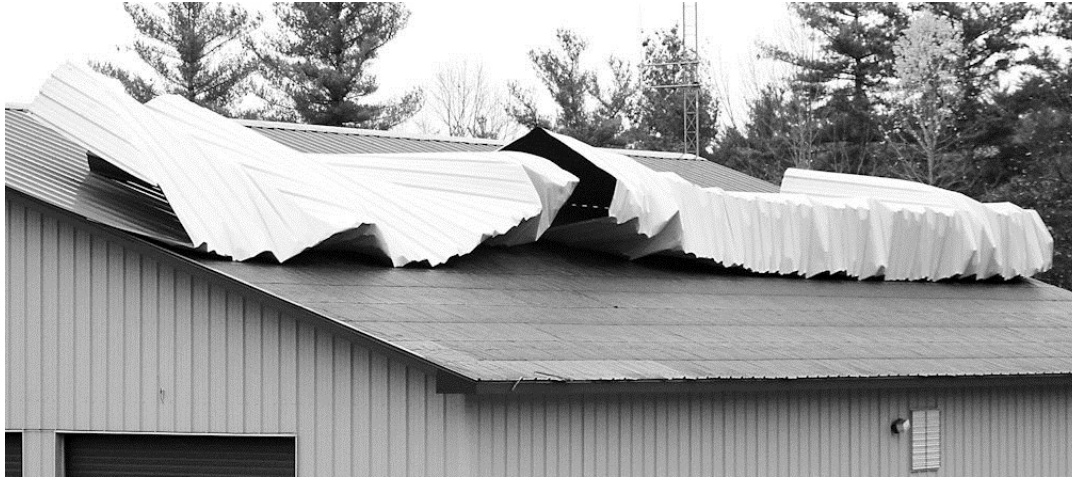
Strong winds Nov. 2 rolled up the roof over the fire station. All of the metal roofing on the north side had to be removed. The project was completed Dec. 5.
