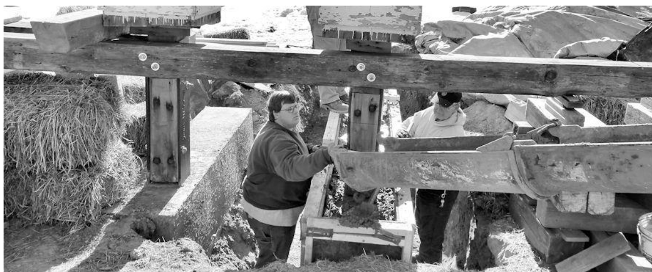
James Long and sons poured concrete Feb. 10 for one of two outside supports under the westerly gate. The first pour on the two inside supports was done Jan. 26, seen on the next page.
