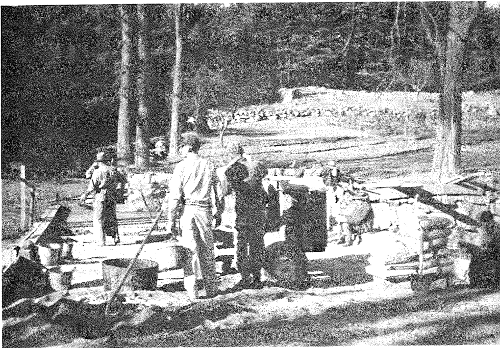
The site first had to be filled with stone before the floor was poured.
