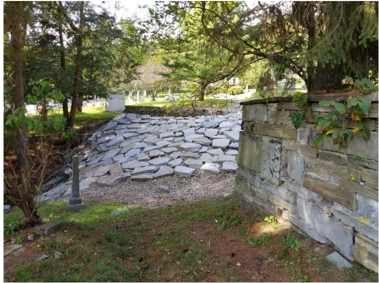
Flat stones have replaced an historic stone parapet-topped culvert.
