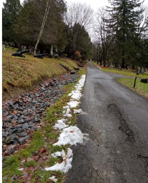
Stone rip-rap has been installed in the grass swales to help intercept runoff from the cemetery's upper slopes.
