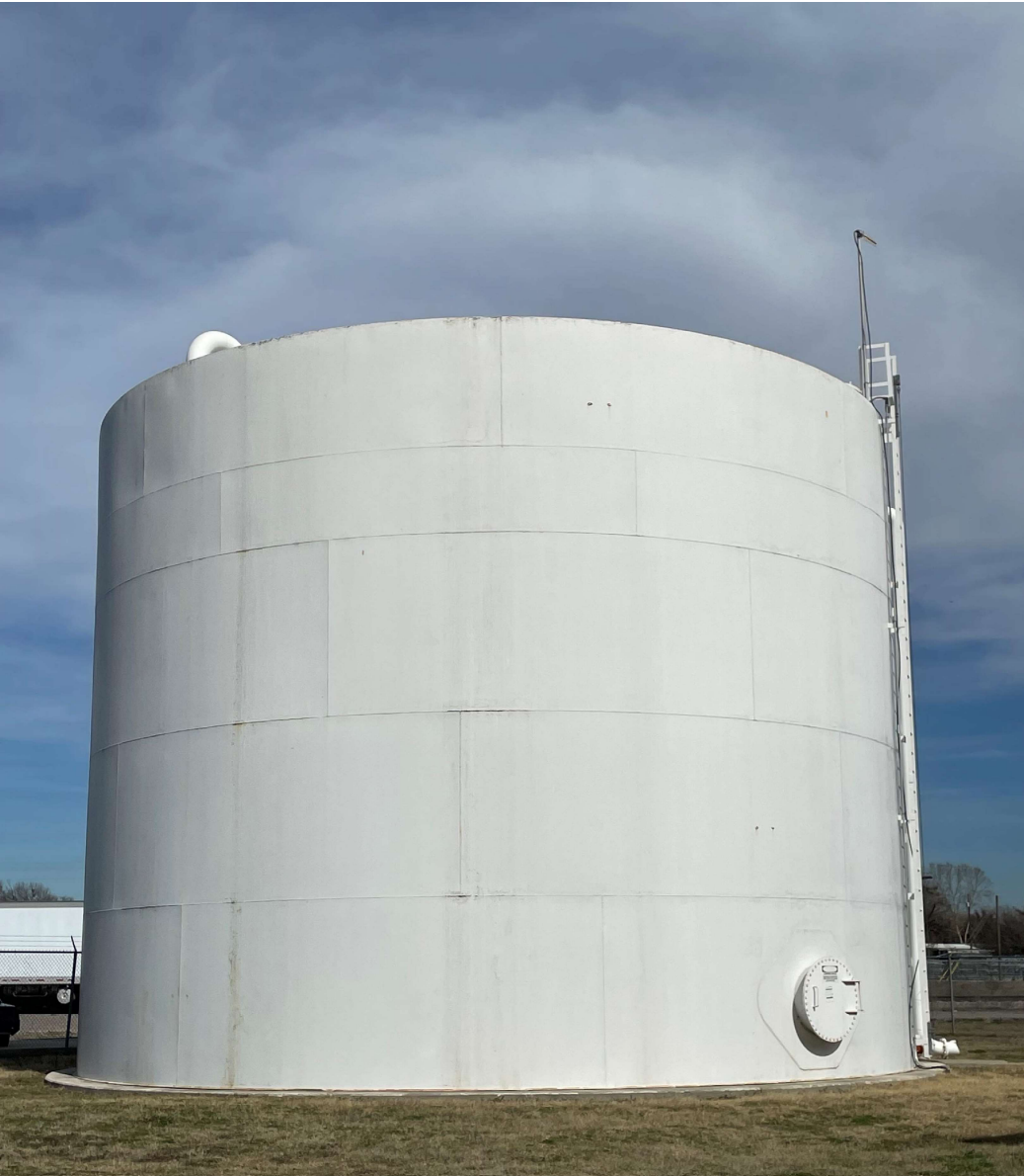
Bobo Pump Station Tank - Exterior
