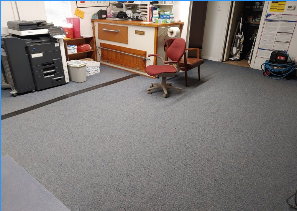
Carpet worn - taped together
