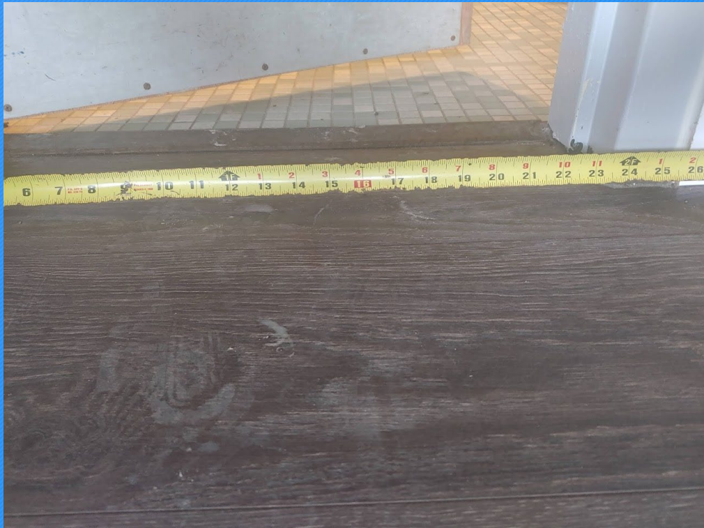
Bathroom doorway not ADA compliant
