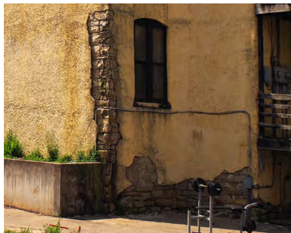
Right: The EFIS on the rear of 525 E Capitol is flaking off.
