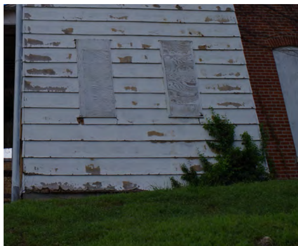
Left: The steps leading to 410 E. Capitol Avenue are sagging, uneven, and deteriorated.
