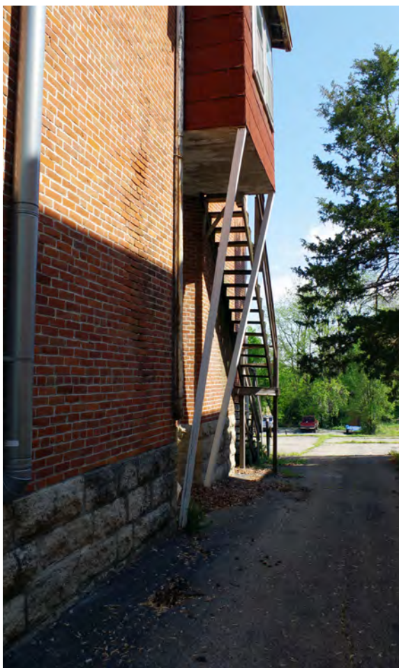
Left: An example of an upper floor exit that is supported by 2x4s.
