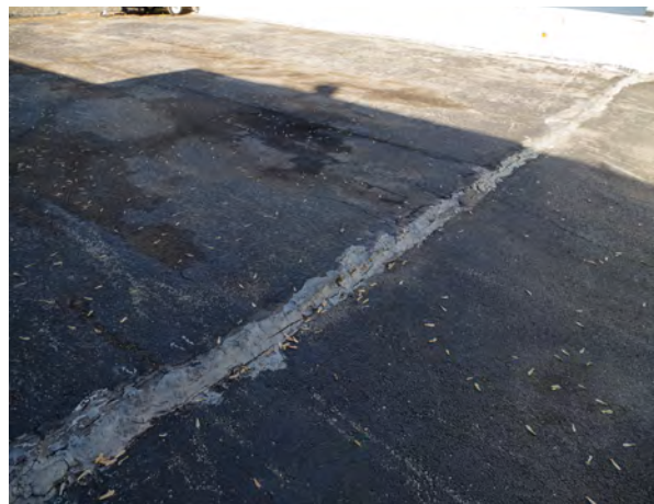
Left & Right: A failing expansion joint on the raised parking lot located at 520 E. High.
