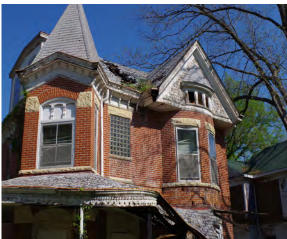
Left & Right: 108 Jackson Street is dilapidated. This vacant home has a collapsed porch, a large hole in the roof, and is boarded-up.
