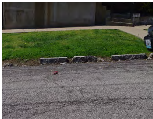
Right: A deteriorated curb and gutter along Marshall.
