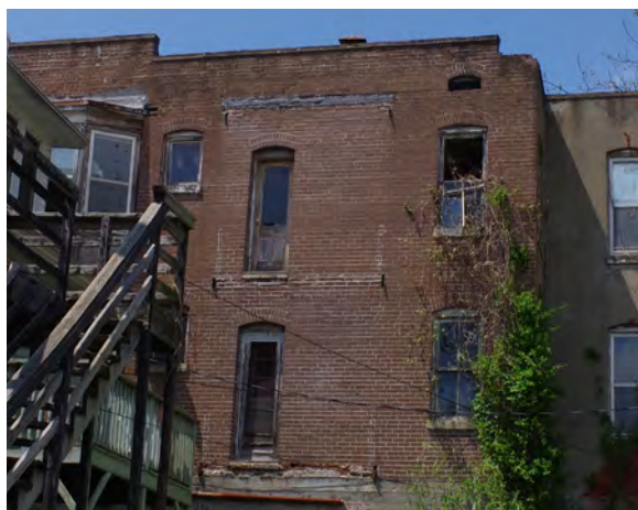
Left: 519 E. Capitol is boarded-up and vacant. The windows, doors, exterior walls, and roof are all severely deteriorated.
