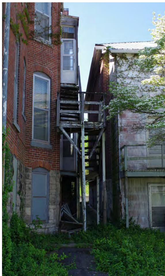
Left: An example of an upper floor exit that is supported by 2x4s.
