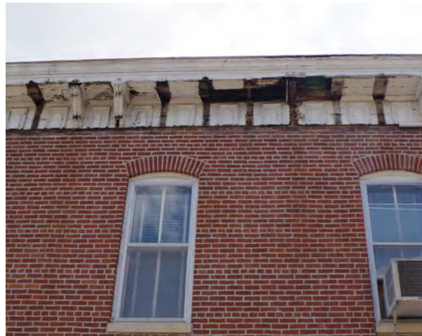
Left & Right: The gutters, downspouts, soffit, and fascia are deteriorated on 507 E. Capitol.
