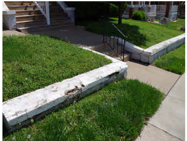
Right: The retaining wall in front of 415 E. High is deteriorated.
