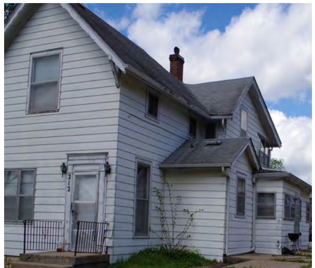
Left: The soffits, fascia, porch, and gutters on 214 Jackson are deteriorated. Downspout is missing.
