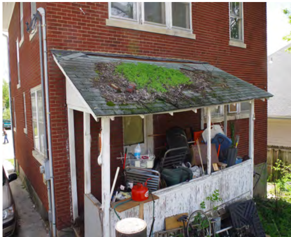
Left & Right: The rear porch, and guttering on 214 Jackson Street are deteriorated.
