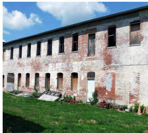
Right: 100 Lafayette is missing the rear windows allowing the weather to penetrate into the structure.
