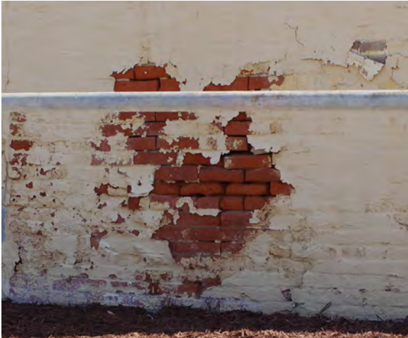
Left: The rear structure at 600 E. Capitol needs tuckpointing.
