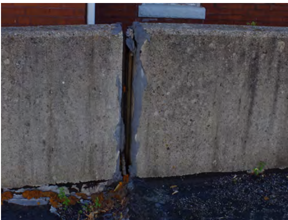
Left & Right: A failing expansion joint on the raised parking lot located at 520 E. High.
