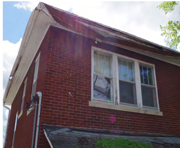
Left & Right: The rear porch, and guttering on 214 Jackson Street are deteriorated.
