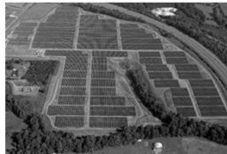
Apple's 100-acre 20 MW facility, Maiden, NC
