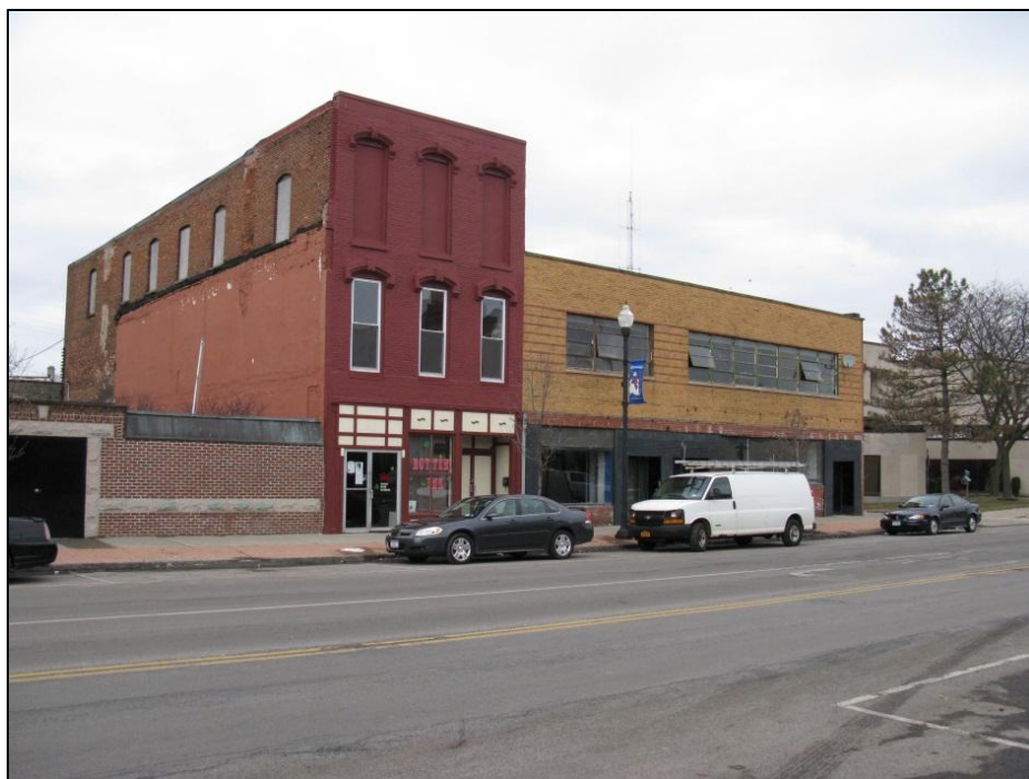
(Above) The three-story Italianate commercial building at 17 West Main Street retains its ornate window surrounds, although the heavy decorative cornice—which was likely constructed of metal—no longer exists.
