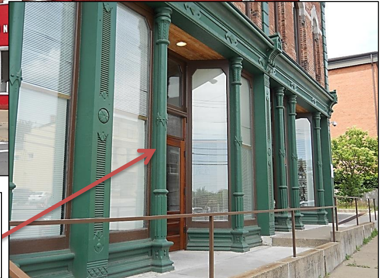
CAST-IRON CORNER PILASTERS FRAMING DISPLAY WINDOWS AND ENTRANCE
