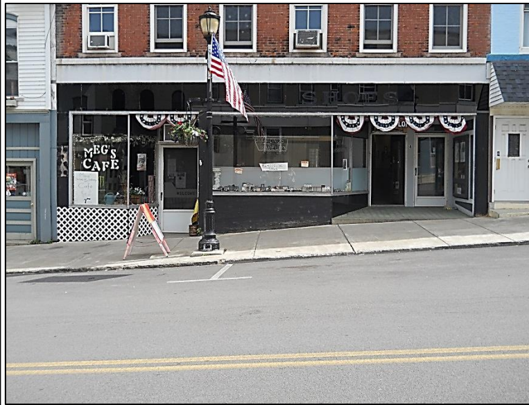
(Left) Decorative cast-iron pilasters, a plain structural beam, and bulkhead, or kick-plate, are architectural elements of this nineteenth century Italianate storefront at 36 Canal Street. (Above) The first-floor at 8 Canal Street features a modern broad-front with a reinforced openness of the façade and recessed entry.
