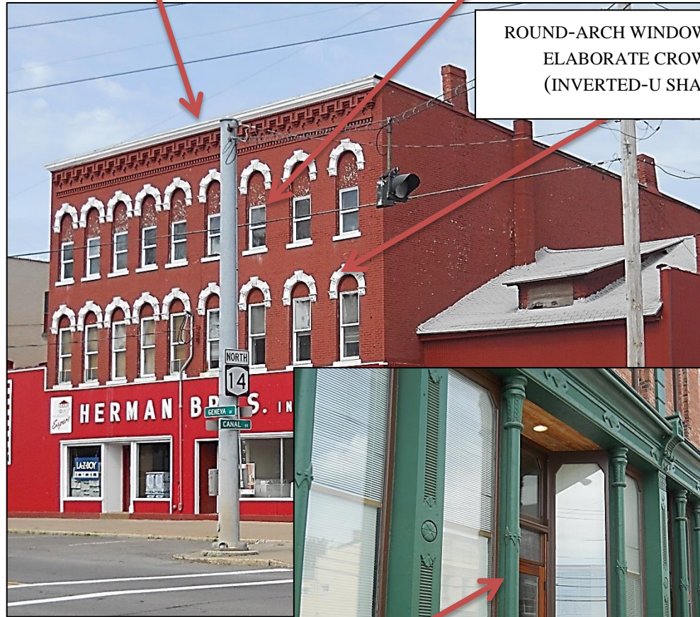
CAST-IRON CORNER PILASTERS FRAMING DISPLAY WINDOWS AND ENTRANCE
