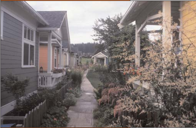
Third Street Cottages with adjacent development in the background
