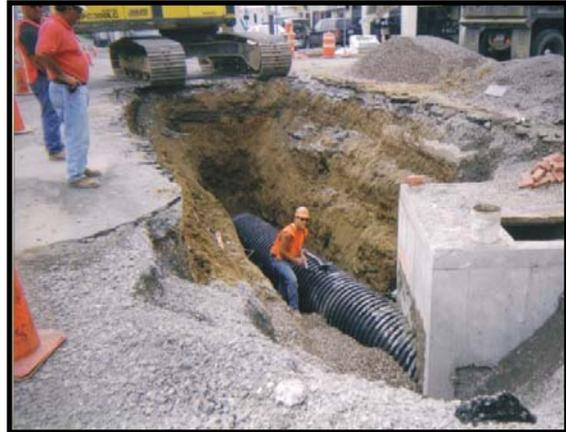
***What Lies Beneath?*** Much can lay hidden beneath the surface, and even the most comprehensive utility surveys can still yield incomplete or inaccurate results. (Pictured: storm and sanitary sewer construction in the Village of Livonia – Photo courtesy of Mayor Cal Lathan).
