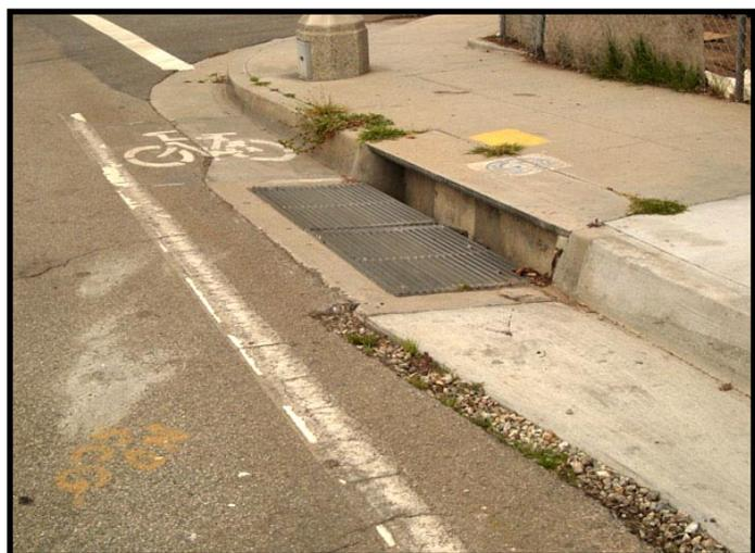
*Safe accommodations for bicyclists should be well-conceived and an integral part of the roadway in order for them to be successful. While the above picture illustrates a desire to accommodate bicyclists, the path provided is full of hazards.*
