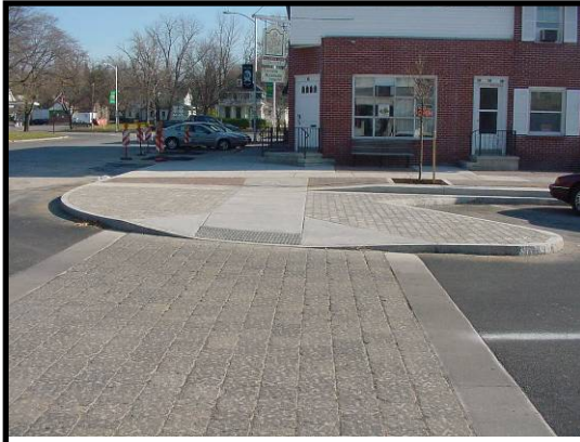
Curb Extension added to Main St. Avon, NY, with inlaid pavers for the crosswalk.
