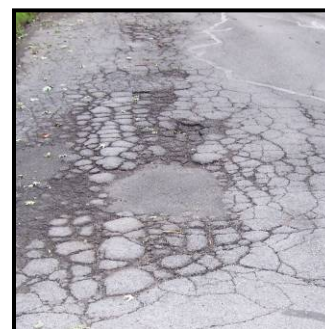
Example of significant alligator cracking with attempts of repair (unspecified location, outside of Scottsville)
