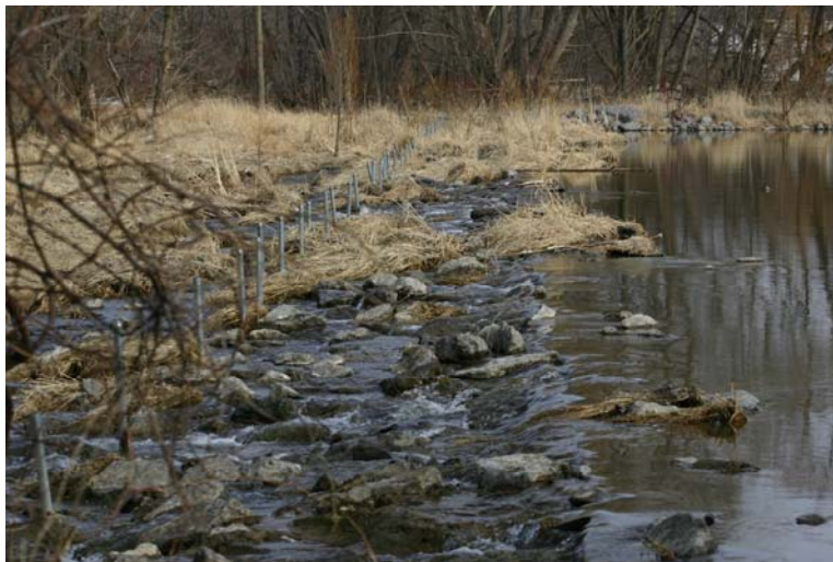
Figure 2-3: Honeoye Outlet Weir
