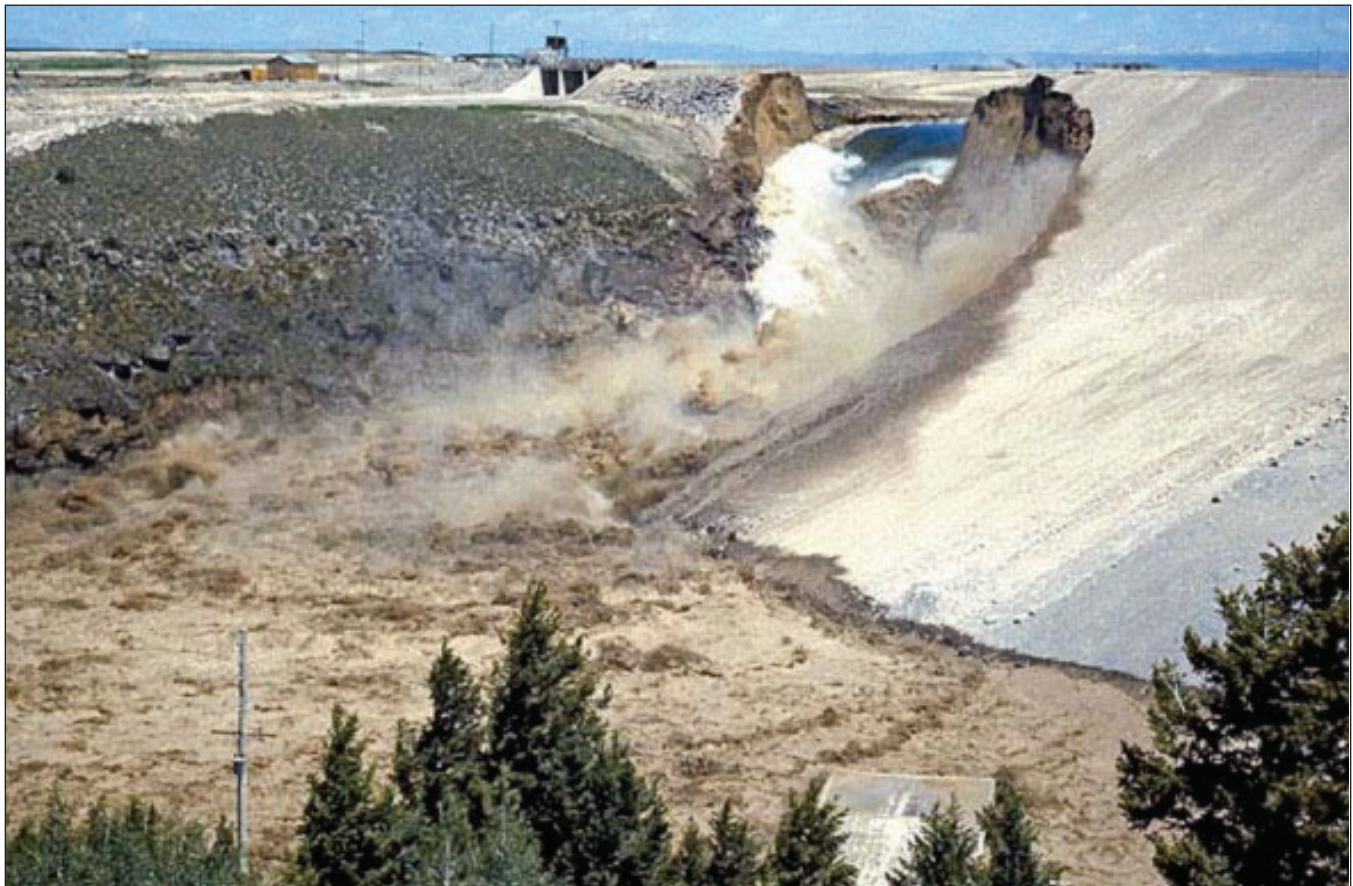
Figure 7-1. Teton Dam Failure, 1976
