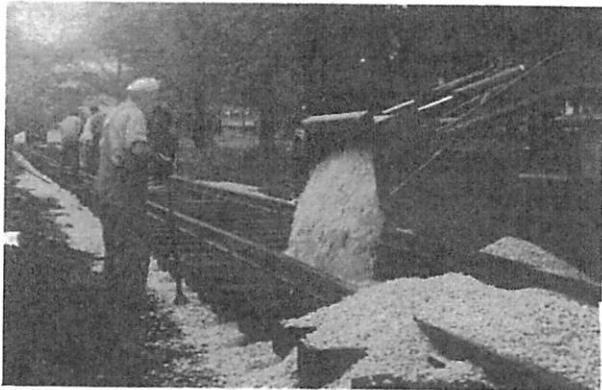
SEPT. 26, 1964 — GRADER DUMPING BALLAST, LOOKING EAST.
