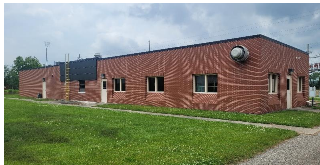
Above: The main building of the Treatment Plant where the lab, office, influent room, pumps, and
