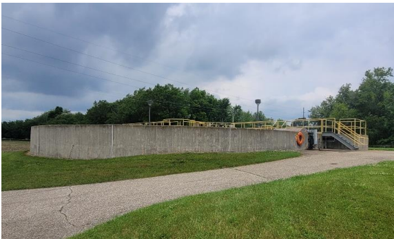
Above: The Wastewater Treatment Plant oxidation ditch which is part of the waste treatment cycle
